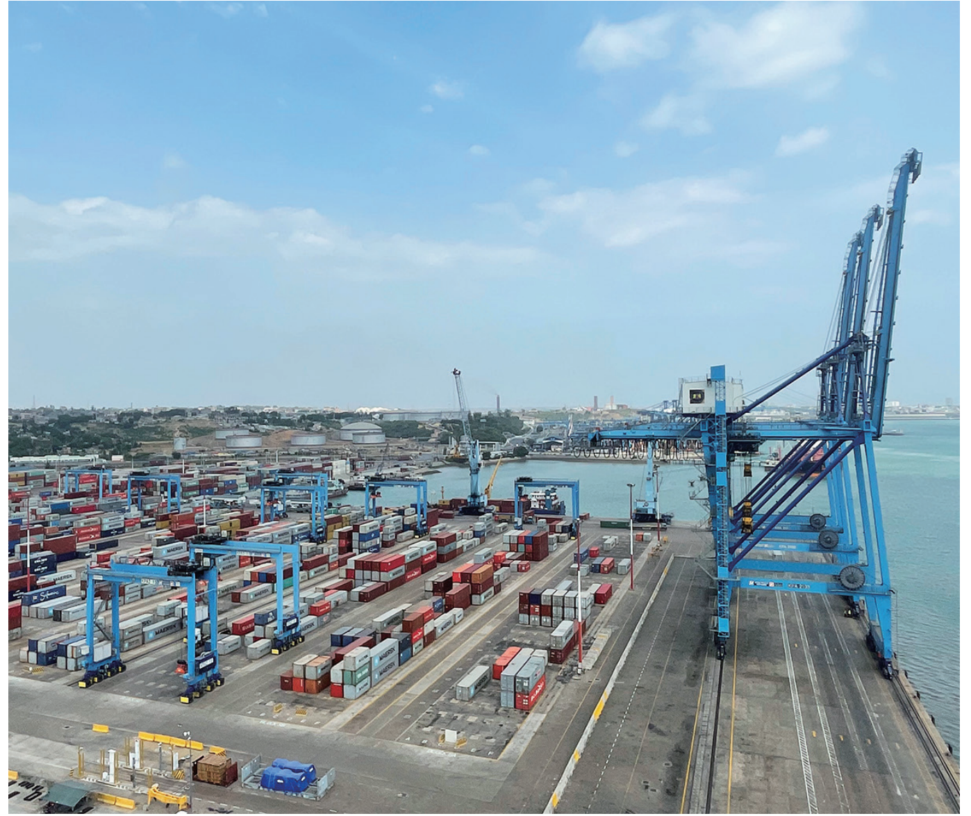
Expansion of the Mombasa Port Container Terminal, a gateway to East and Central Africa
